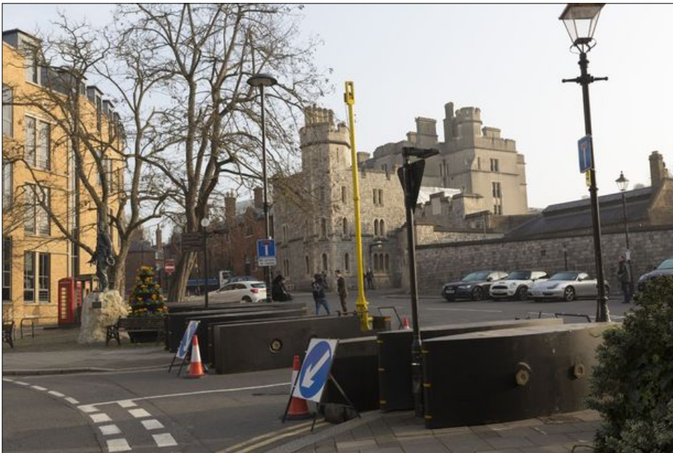
Image 1: Example of temporary NBA measures on Park Street
